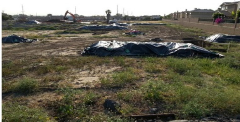
Soil Remediation Underway
