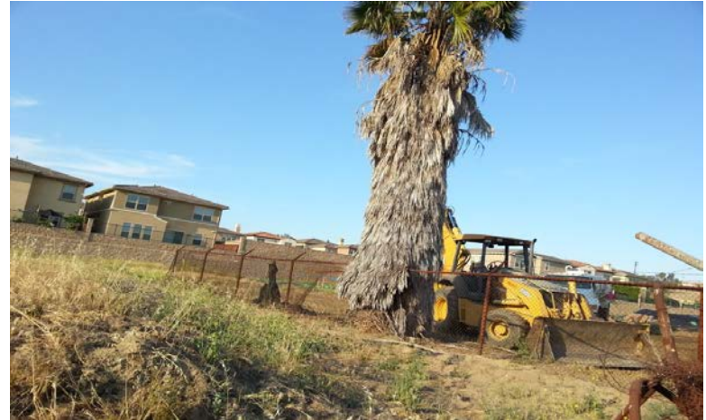
Precise excavating of contaminated soils
