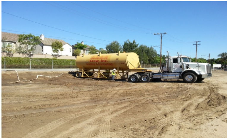
Setting up water tower for dust control
